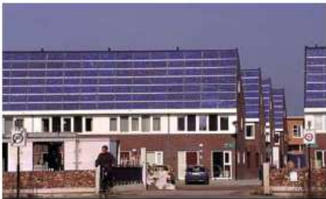
Figure no.6: Building Integrated (BIPV) in the Netherlands
