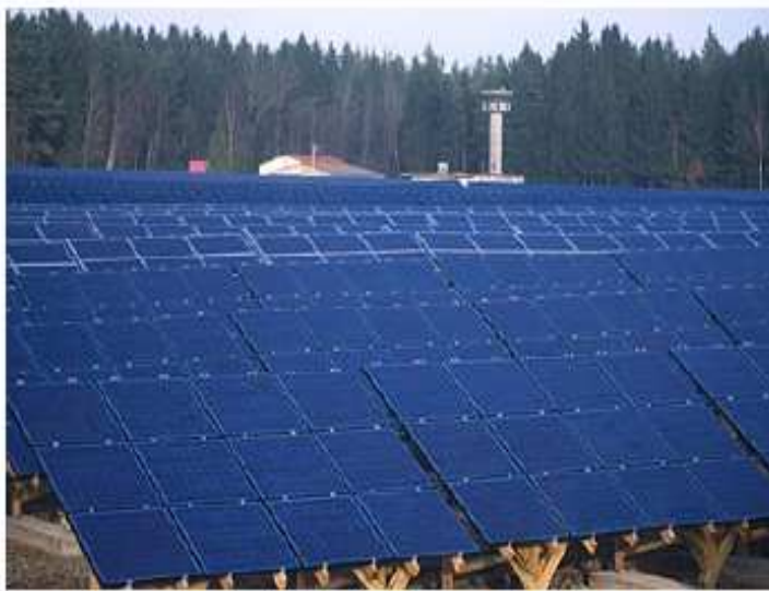
Figure no.5: 7MWp Solar Power station in Germany
